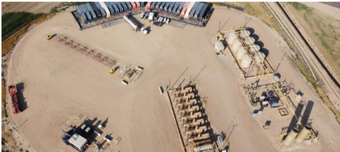
Figure 37: Aerial photo of Bayswater's temporary water treatment facility located on an existing Bayswater production facility in Weld County, Colorado. Produced water was being treated in the tanks at the top of the photo, recycled to be used in completion operations, and then transported to wells being hydraulically fractured via poly pipe.
