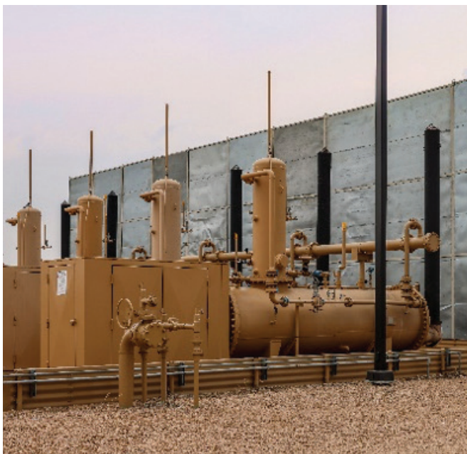
Figure 39: Photo of a permanent sound wall Bayswater erected at a production location to minimize noise impacts to nearby landowners.
