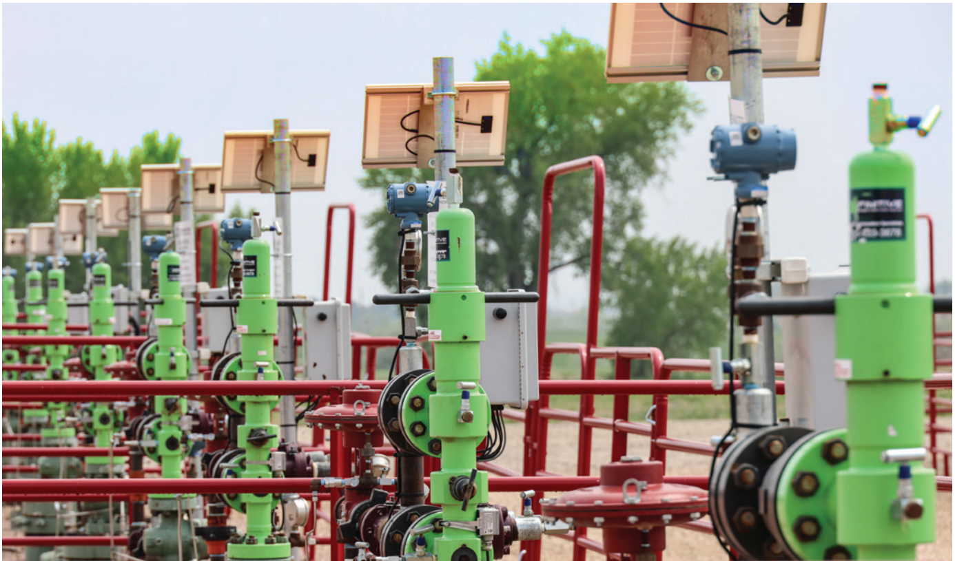
Figure 33: An example of Bayswater utilizing solar arrays to help power wellheads on a Colorado production site.
